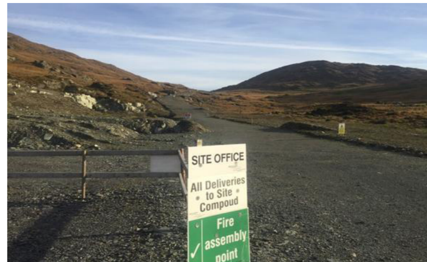
View of civil works at site entrance
