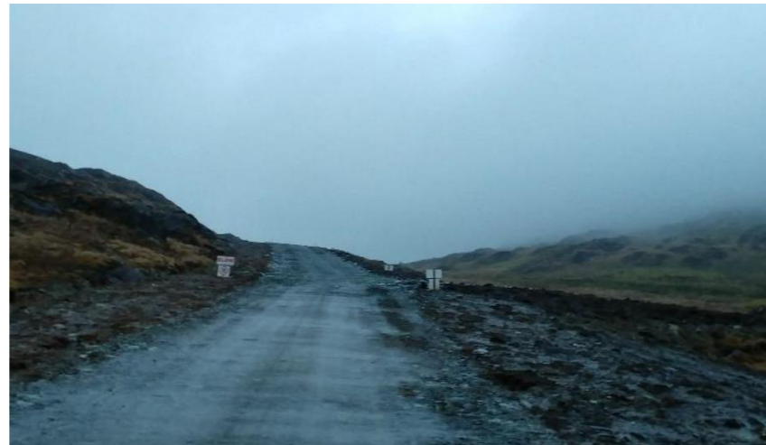
View of site track towards the east
